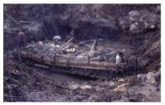
Figure 2: In order to extract the wreck from the silt of the river, it was required to detach it from the ground by creating a platform of horizontal tubes
