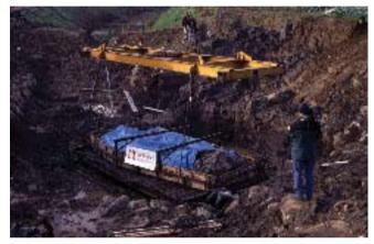
Figure 3: Once detached from the silt, it required a large crane to lift the block of the wreck onto the bed of a special truck of adjustable height
