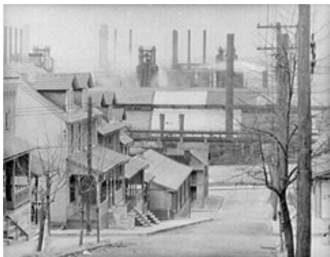
Bethlehem Steel Plants, historic view
