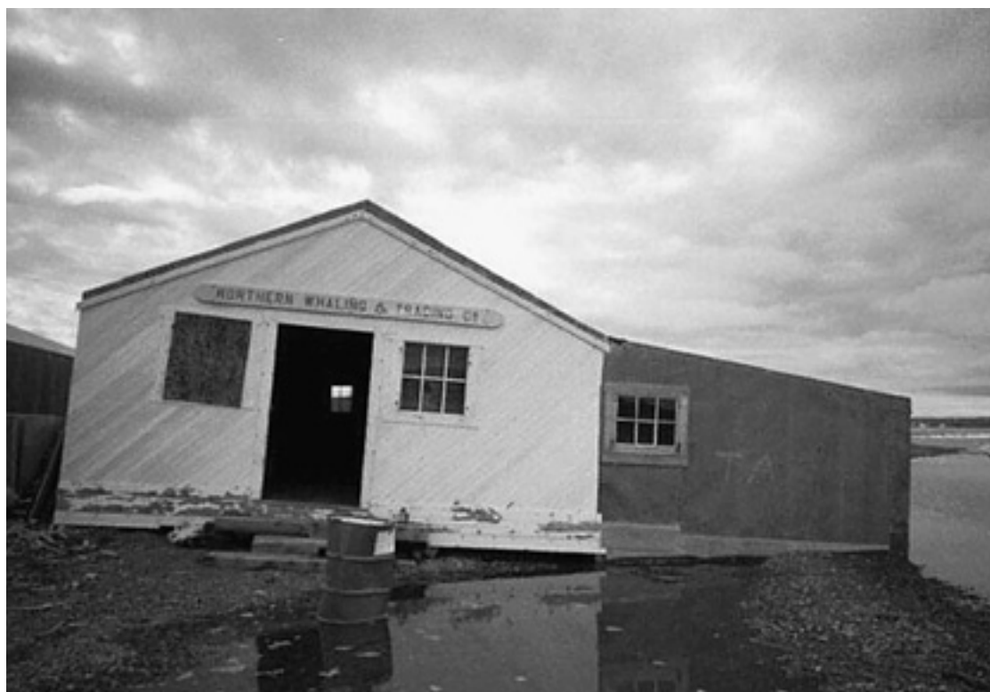
Northern Whaling and Trading Company Store, Pauline Cove, Western Canada Arctic, prior to dismantling of shed addition in 2000
