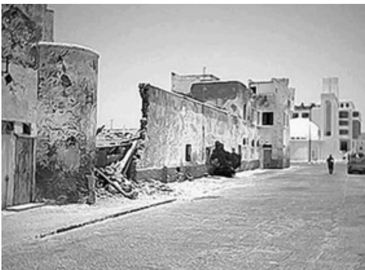
Demolition of a wall of the fort
