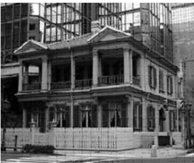
Kyokoryuti 15 banken, in process of reconstruction
