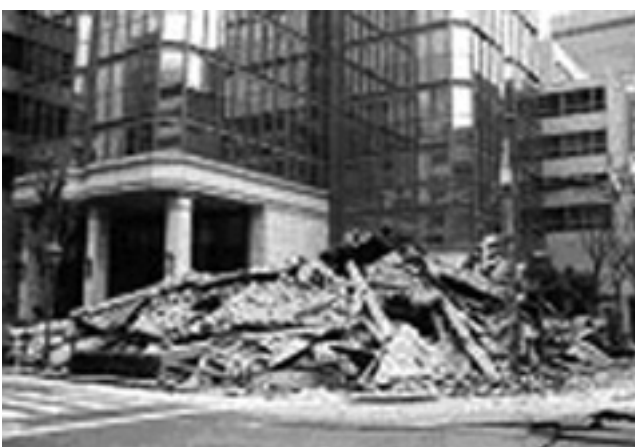
Kyokoryuti 15 banken, destroyed by earthquake
