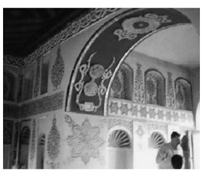
Walls are thick, built of stone and plastered with lime mortar. Roofs are of mud carried on woven mats placed above wooded joints. Windows are small and directed towards the prevailing breeze. These features provide thermal comfort without recourse to electricity.
