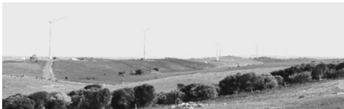
Wind Farm near Codrington in Western Victoria (photo: Codrington Wind Farm Tours http://www.myportfairy.com/windfartours )
