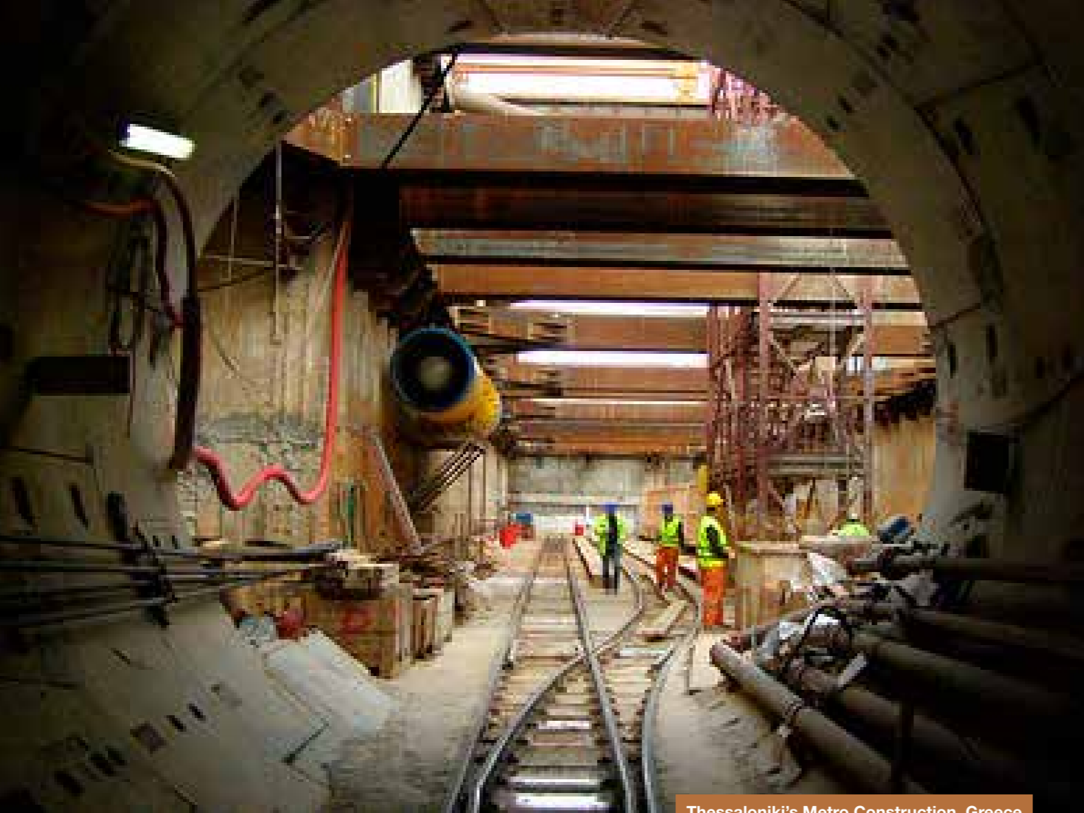
Thessaloniki's Metro Construction, Greece
